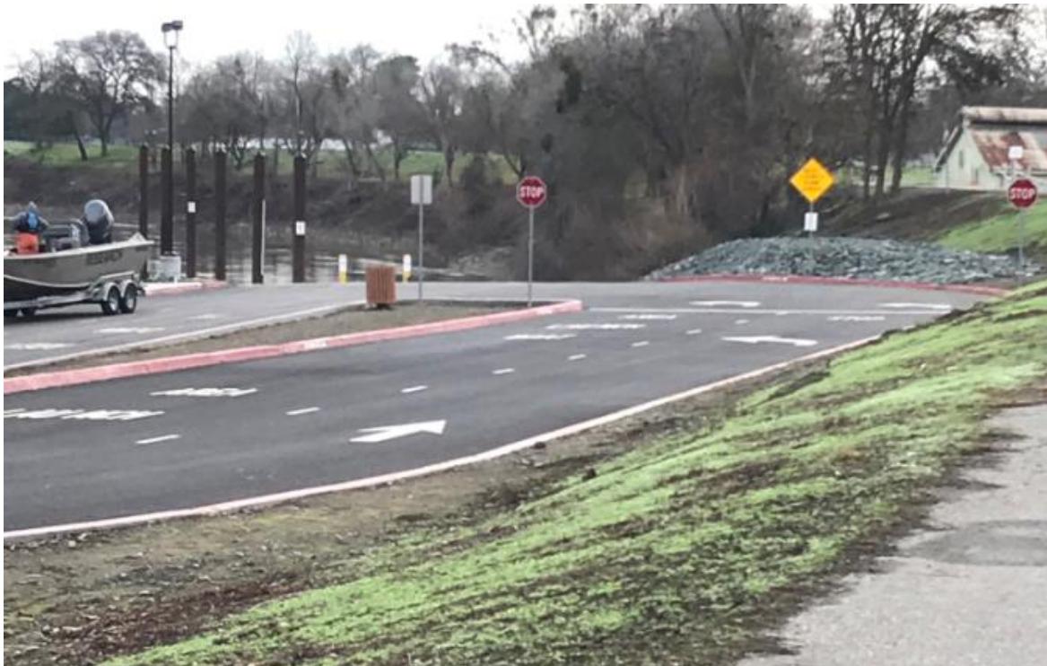
Access roadway to ramp
