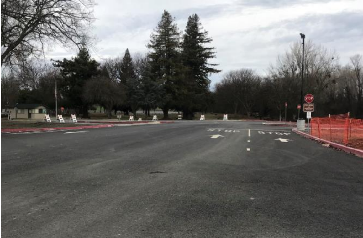
Boat Launching Facility entrance roadway
