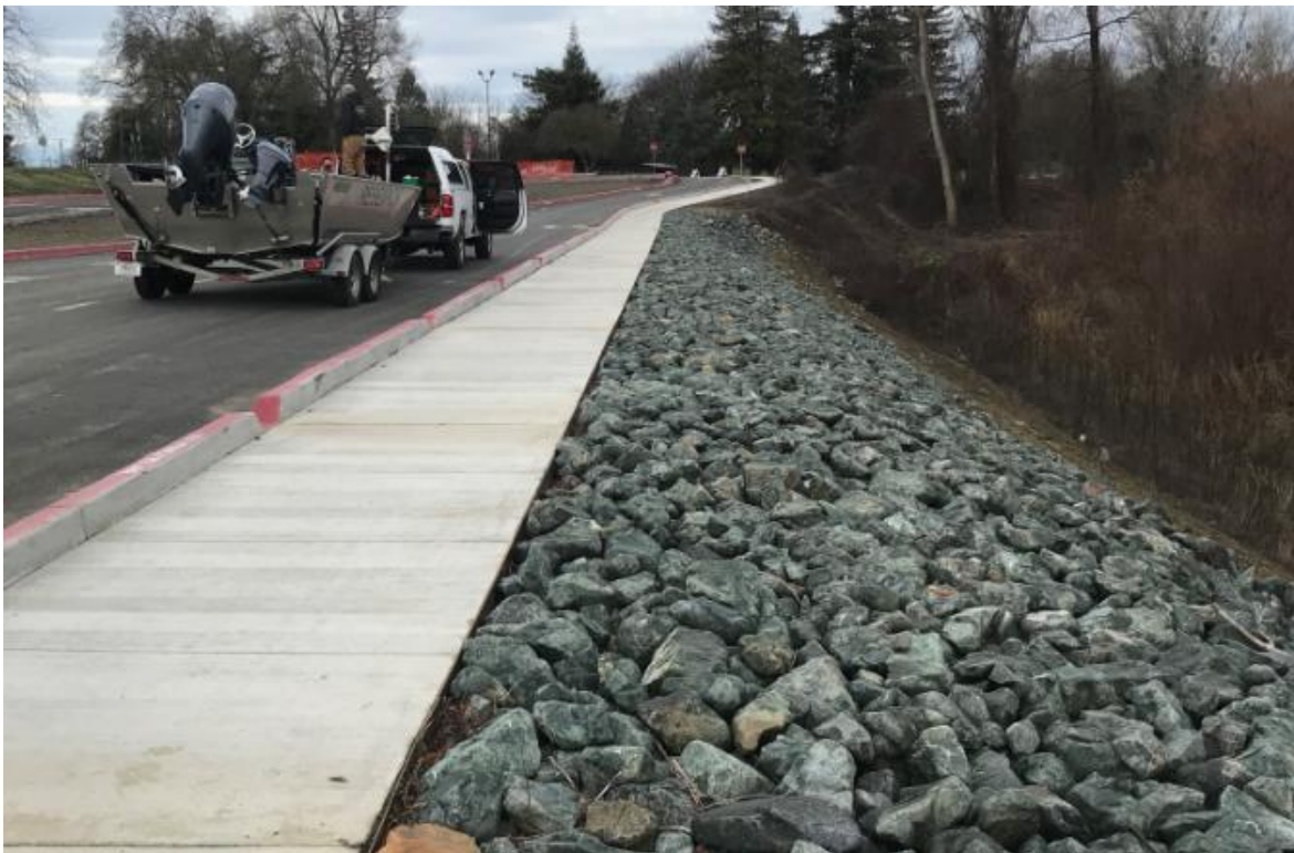
Accessible pathways and slope protection
