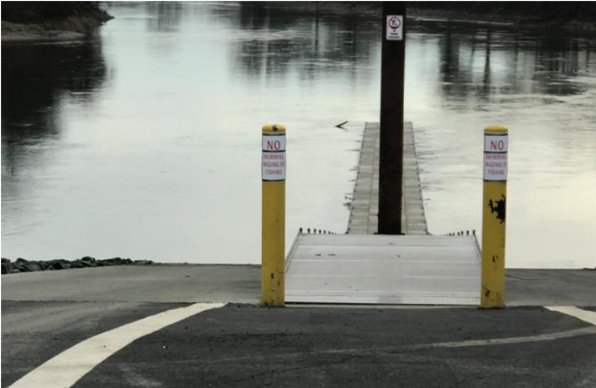
Boat ramp and pile-guided boarding float
