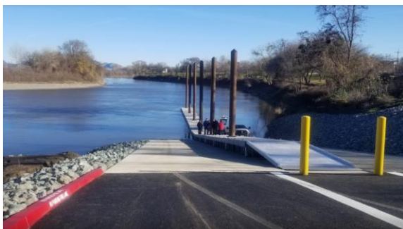
Top of the boat ramp
